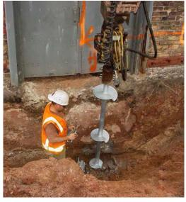
different helical pile designs for each side. In addition, some soil boring logs reported very soft clay between 35 to 50 feet below grade and to beyond the boring depths.
