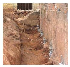
Installation torsion on a helical pile shaft is an indication of the ultimate capacity of the pile. The 2-7/8 inch diameter piles were installed to torques between 5,000 and 10,700 ft-lb with the larger torsion readings generated from the piles encountering cemented sands.
