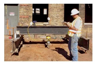
This concern materialized when pile numbers 23 and 24 achieved suitable torsion only after reaching depths of 92 feet and 87 feet respectfully. Specific concerns about the strength of these piles were satisfied by Lipe Brothers Construction. After installation, these piles were test loaded to 62,000 pounds and monitored for creep over a period of 80 minutes. Once accomplished, suport was verified and the engineer approved the piles.
