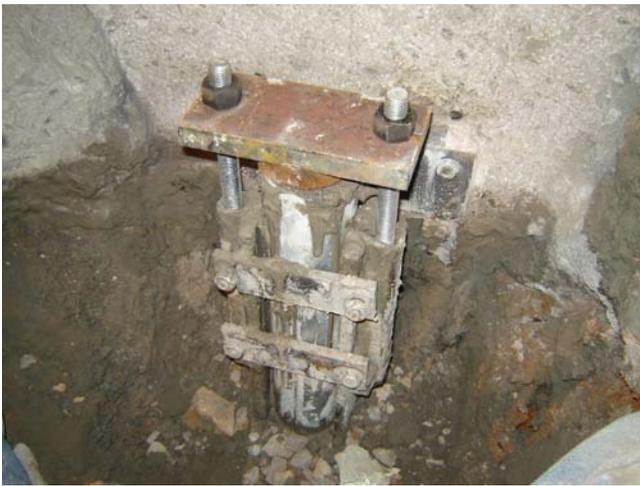
After the grout achieved the design compressive strength of 4000 psi, the micropiles were loaded to 17,000 pounds and locked off within the brackets. This transferred 90% of the wall load to the micropiles. The gap between the wall panels and the footing was filled with grout to completely transfer the load to the micropiles.
