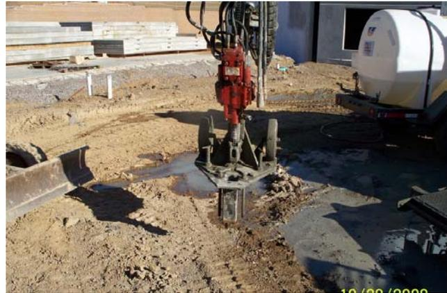
Foundation Specialties, Inc. was retained to perform emergency remedial underpinning at the Fort Smith Pavilion. Several precast tilt-up panels with integral columns placed on spread footings with column pads had been damaged when the footings settled during construction.
