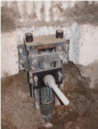
installed the pier driving equipment against the wall. Notice that the footing has been carefully notched to place the pier bracket under the structural wall. The final configuration of ECP Steel Pier™ and Torque Anchor™ tieback is shown left.
