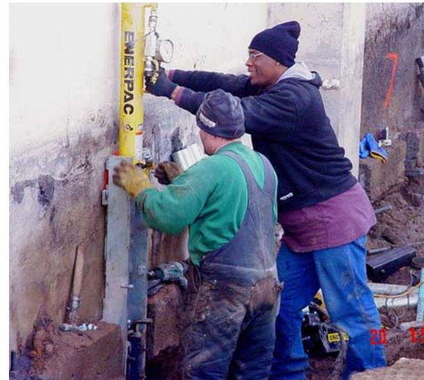
The photo at upper right shows a hydraulic motor installed on a backhoe being used advance a Torque Anchor™ tieback under the structure. Once accomplished, technicians
