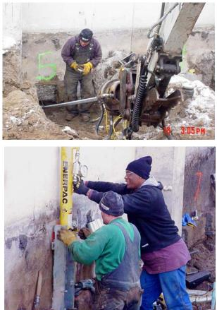
installed the pier driving equipment against the wall. Notice that the footing has been carefully notched to place the pier bracket under the structural wall. The final configuration of ECP Steel Pier<sup>™</sup> and Torque Anchor<sup>™</sup> tieback is shown left.
