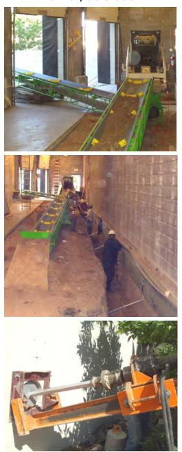
From the top: Soil removal was accomplished by conveyor as workers dug behind the stem walls. A helical tieback is installed at the specified angle.
